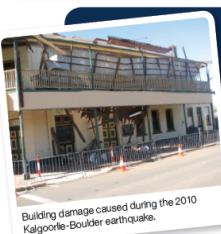
Building damage caused during the 2010 Kalgoorlie-Boulder earthquake.
